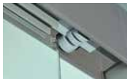
2 Sensors for detector of sash position
